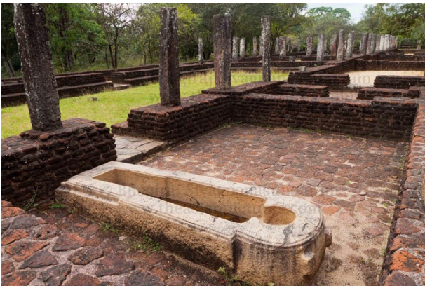
Figure 4. Alahana Parivena hospital complex at Polonnaruwa (12 th century) has been restored by the Cultural Triangle in 1982
